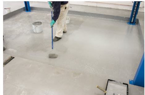
Roller application is quick and easy and gives a good finish.
