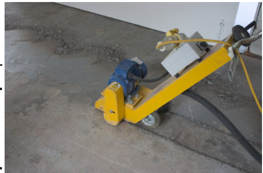
Use a scabbler to remove old coatings and weak concrete
