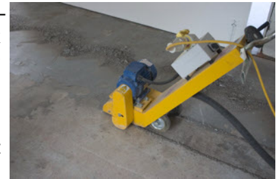
Use a scabber to remove old coatings and soft concrete.
